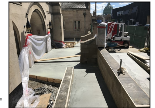
Whitfield St. entrance under construction
